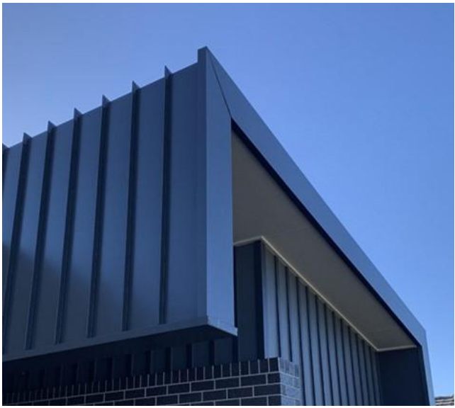
Roofing and Barge Cladding - Lysaght Enseam Colorbond 'Monument' Sheeting Capping and Trim
