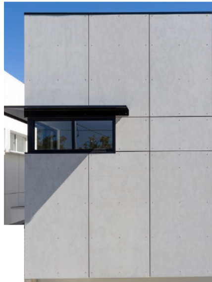
First Floor Walls - FC: CSR Cemintel to match the Existing Adjacent TAFE Connected Learning Centre
