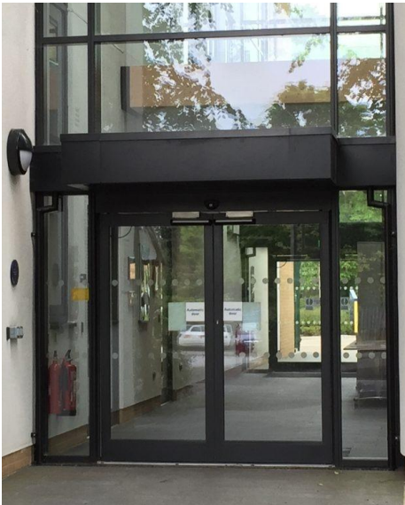
Aluminium Window & Door Framing - WS: Black Powder Coated with Grey Tint Glazing
