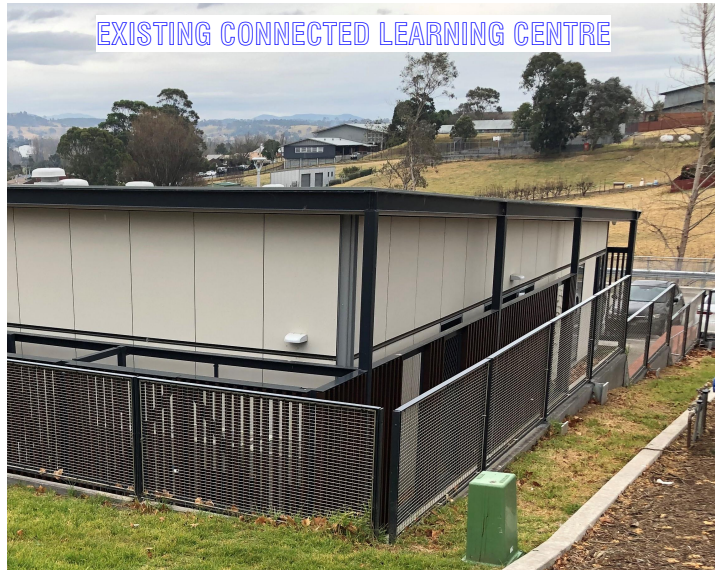
First Floor Walls - FC: CSR Cemintel to match the Existing Adjacent TAFE Connected Learning Centre
